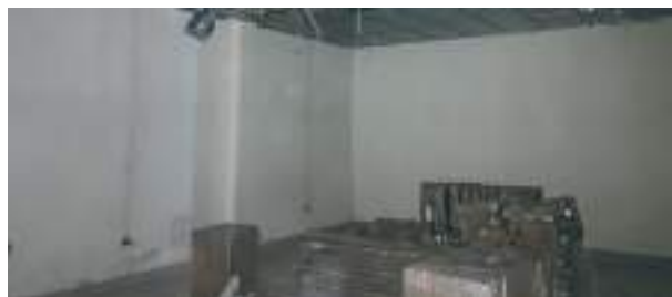
Gedung Lecturer Building - Ruang Kelas Lantai 2
