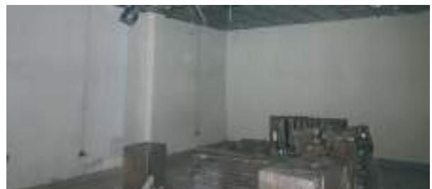
Gedung Lecturer Building - Ruang Kelas Lantai 2
