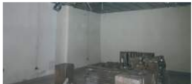
Gedung Lecturer Building – Ruang Kelas Lantai 2
